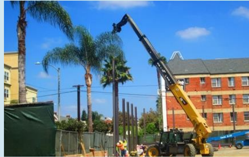
Soundwall Construction at North Wilshire/La Brea
