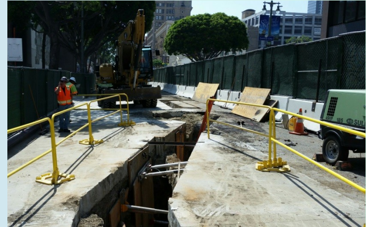
2 nd /Broadway intersection Partial Closure
