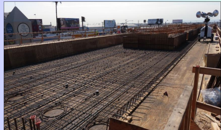
AVIATION/CENTURY BRIDGE – Rebar Installation
