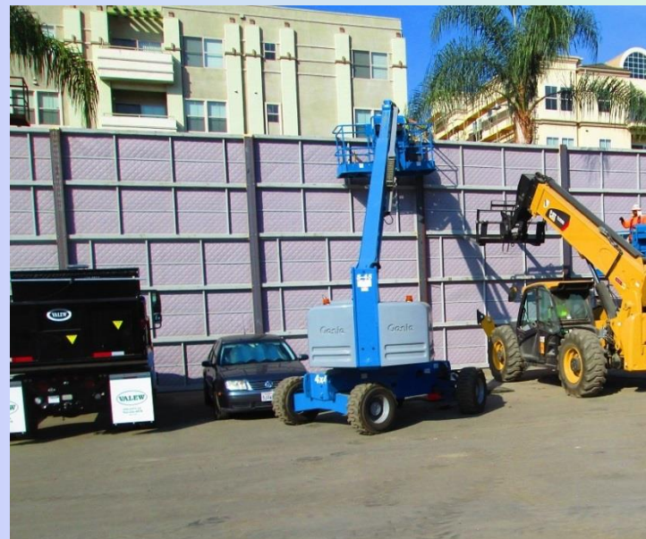
Installation of Soundwall Panels at North Wilshire/La Brea Construction Staging Site
