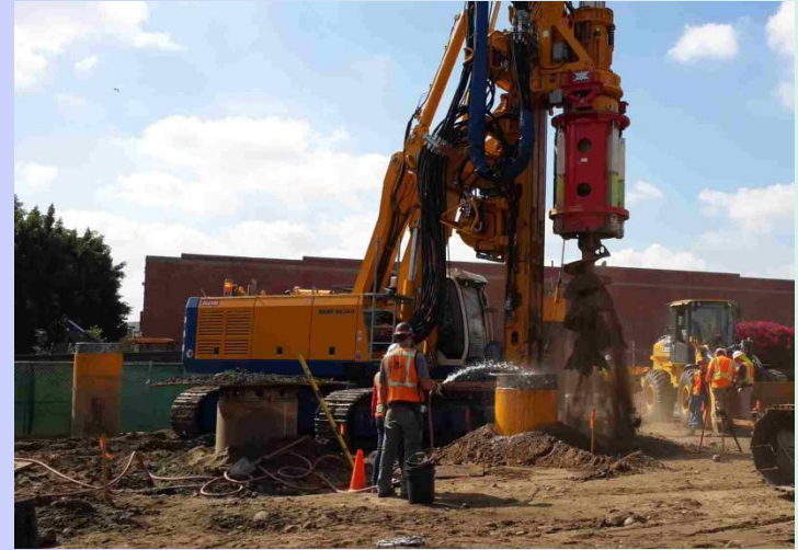
Pile drilling at 1 st /Central Station yard
