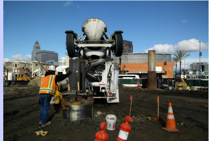
Soldier Pile Installation at 1 st /Central Station
