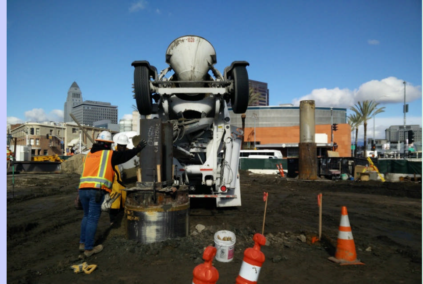
Soldier Pile Installation at 1 st /Central Station
