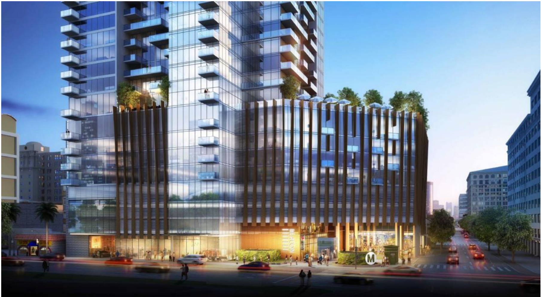
Depiction of Proposed EQR Project (with Building Overhang over Metro's Portal Property)
