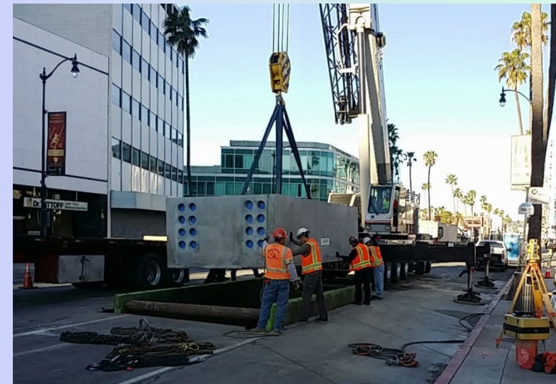
AUR Contractor Installing SCE Electrical Vault West of La Cienega Boulevard
