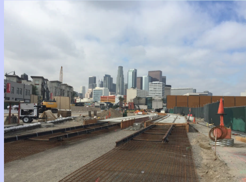
Shoofly installation at Mangrove Yard
