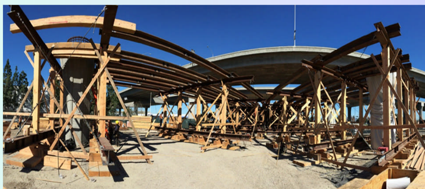
Crenshaw tie-in with Green line falsework construction
