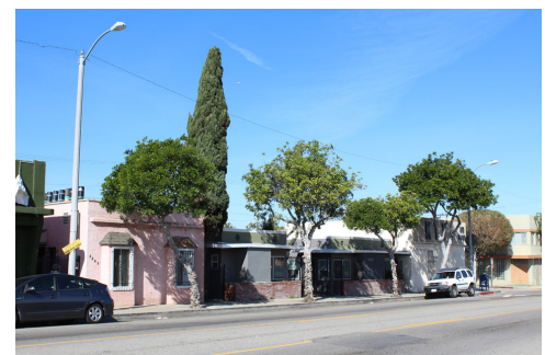
Figure 11 View north along West Boulevard
