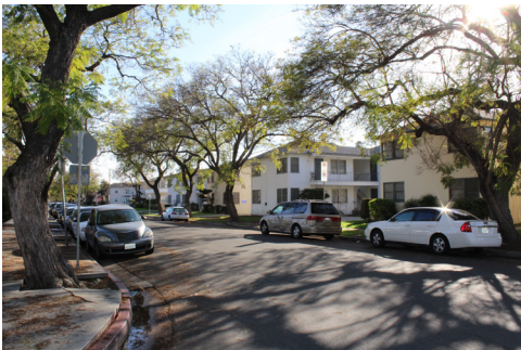
Figure 13 View south along Victoria Avenue
