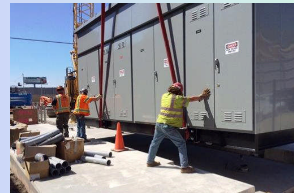
Electrical Metering Switchgear for Tunnel Operations
