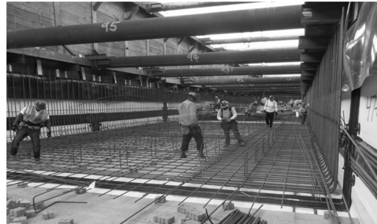
U-Wall and invert rebar installation continues at UG1.
