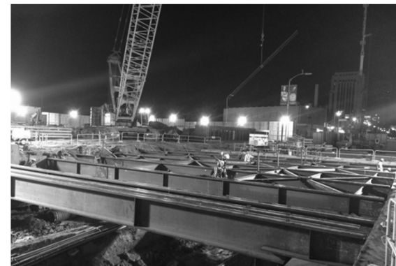
Installation of Deck Beams on Wilshire Blvd.
