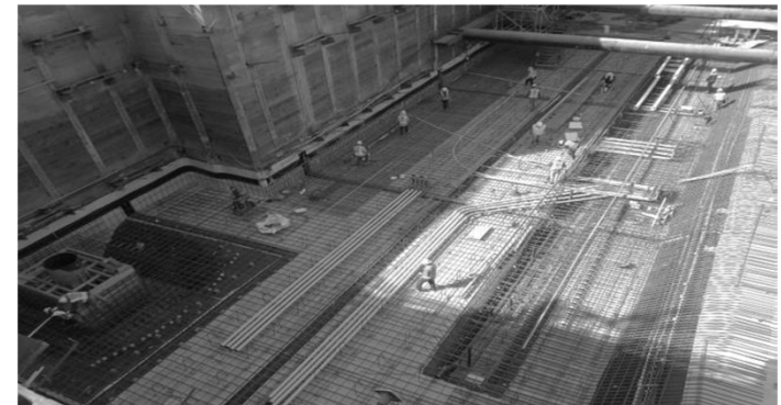
Installation of bottom mat of rebar in 1 st /Central station invert
