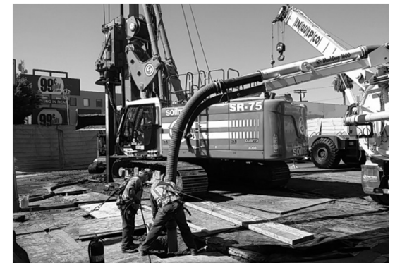
Pile installation activities at Wilshire/Fairfax Station
