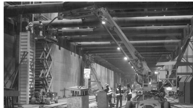
Concrete placement for columns in Expo Station
