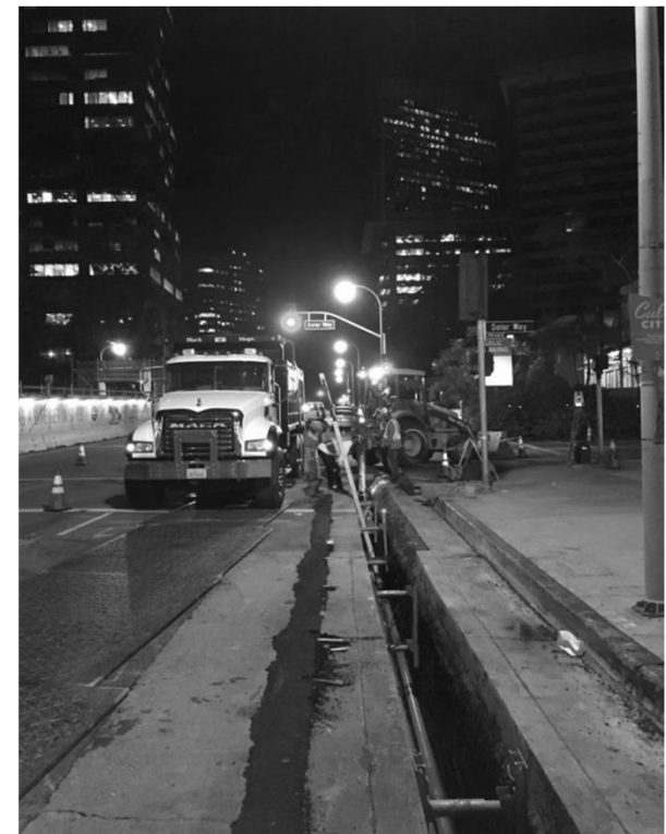
Telcom joint trench construction in Constellation Boulevard
