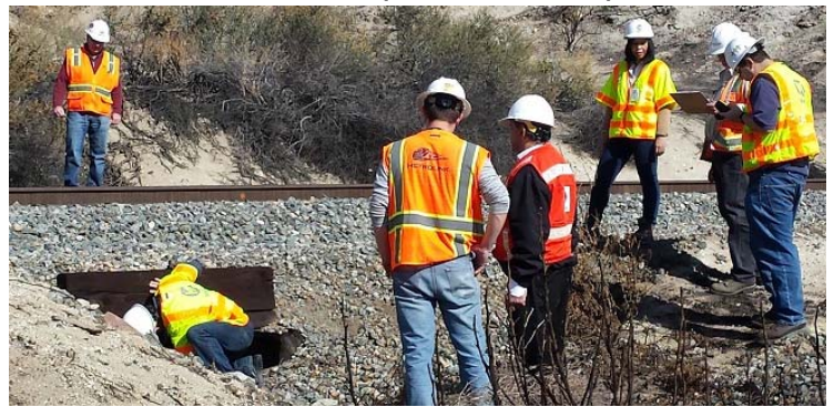
Picture 2: SCRRA Staff and MTA Staff Inspecting a Wood Box Culvert on the Valley Subdivision
