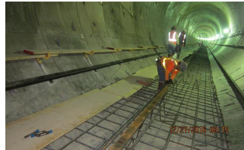
Initiating southbound tunnel concrete invert work
