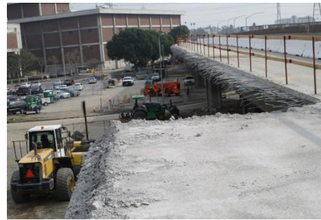
Edge of Deck Removal
