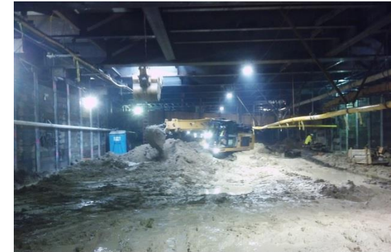
La Brea Station excavation under the deck panels
