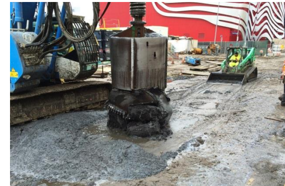
Drilling Piles near Wilshire and Fairfax
