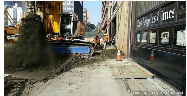
Piling on 2 nd Street (2 nd /Broadway Station)
