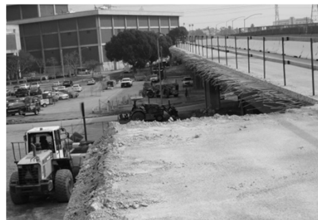
Edge of Deck Removal
