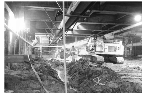
Excavation at Wilshire/La Brea Station
