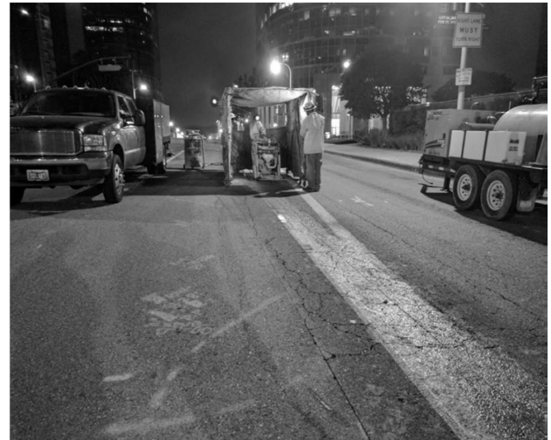
Telecom Joint Trench Construction along Constellation Boulevard
