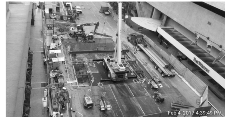
Installation of deck beams on Flower Street
