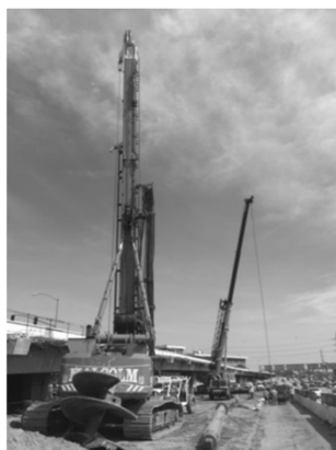
First pile drilling
