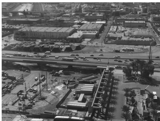
Aerial view of site
