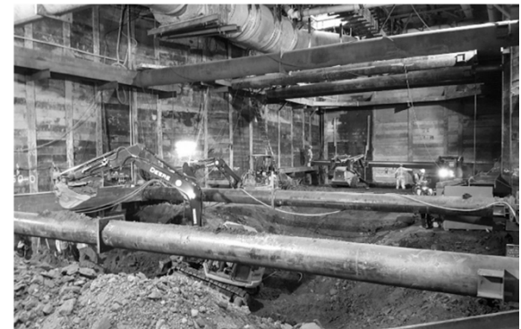
Excavation and lagging for TBM Retrieval Shaft
