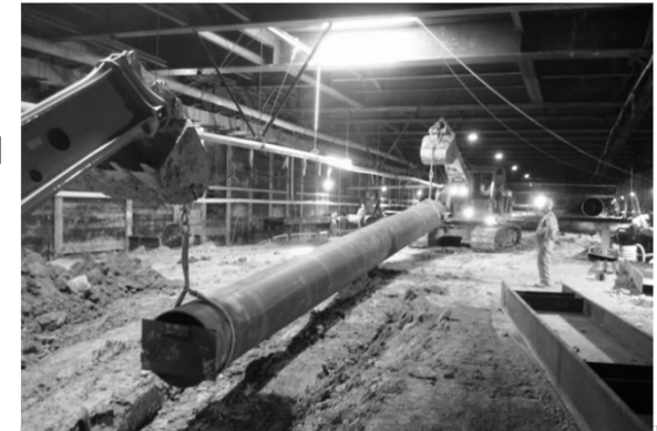
Installing Strut at Wilshire/La Brea Station
