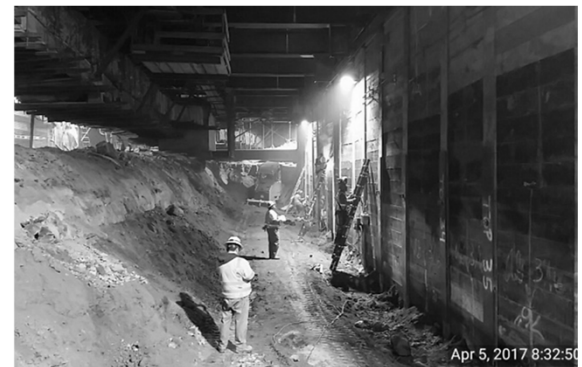
Excavation and utility hanging under 2 nd Street
