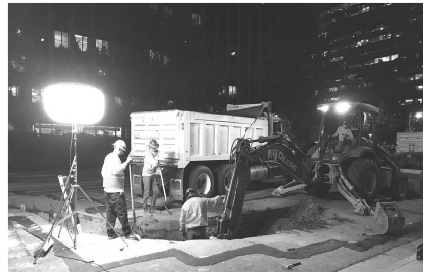
Telecom Joint Trench Construction along Constellation Boulevard
