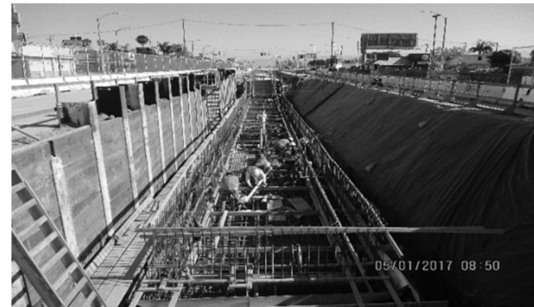
Installation of form work for TC&C room at Hyde Park Station.
