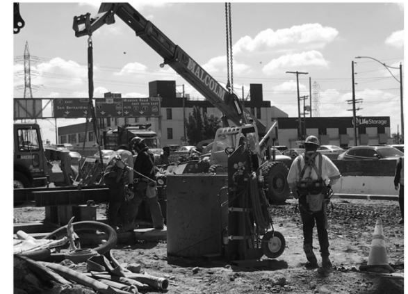
Setting and Pouring Bent 4
