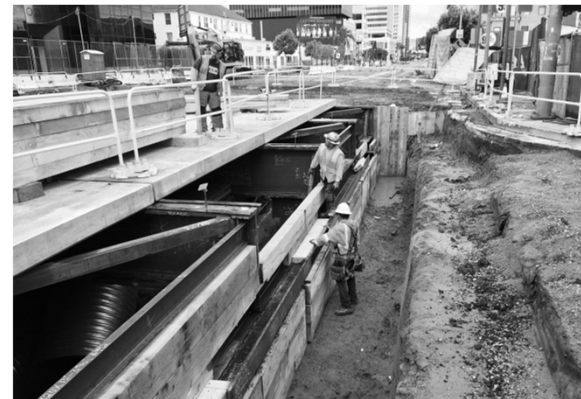
Decking Operation at Wilshire/Fairfax Station
