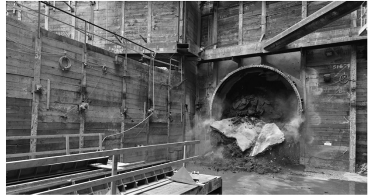
TBM breaking through Grand Av Arts/Bunker Hill Station
