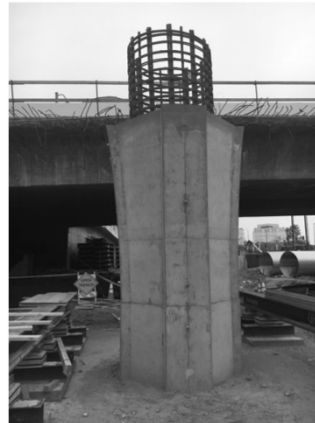
Completed bridge column
