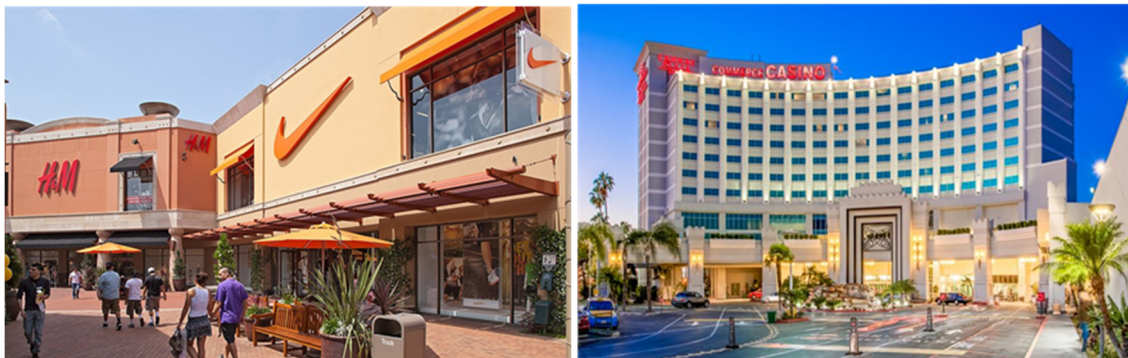
Figure 0-5: The Citadel Outlets & Commerce Casino
