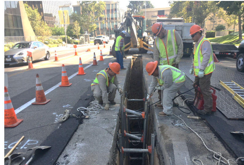
LADWP power relocation work in Century City
