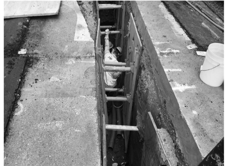
LADWP power relocation work in Century City
