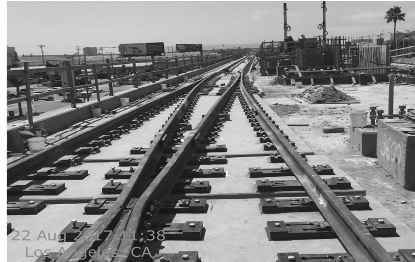
Switch for crossover at Aviation/Century Bridge.
