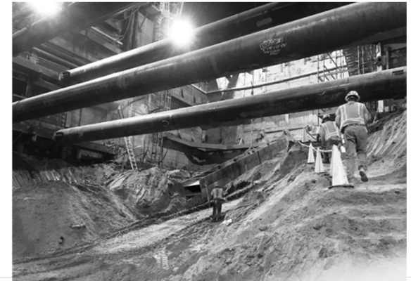
Under Deck Excavation at Wilshire/La Brea Station
