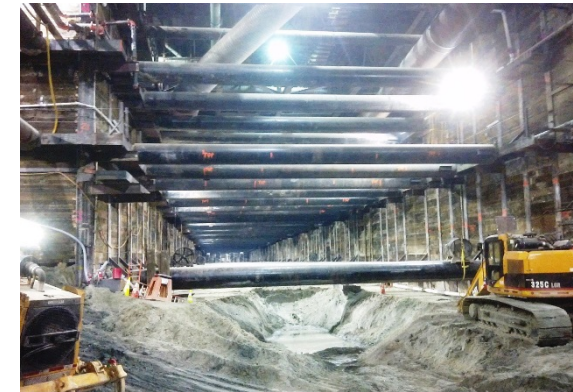
Under Deck Excavation at Wilshire/La Brea Station
