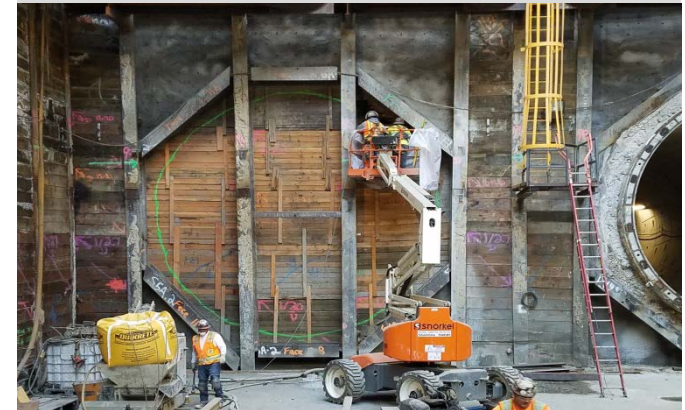
Preparation for shotcrete application at Grand Av Arts/Bunker Hill Station
