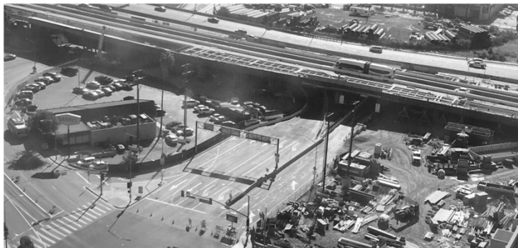
Aerial view of site
