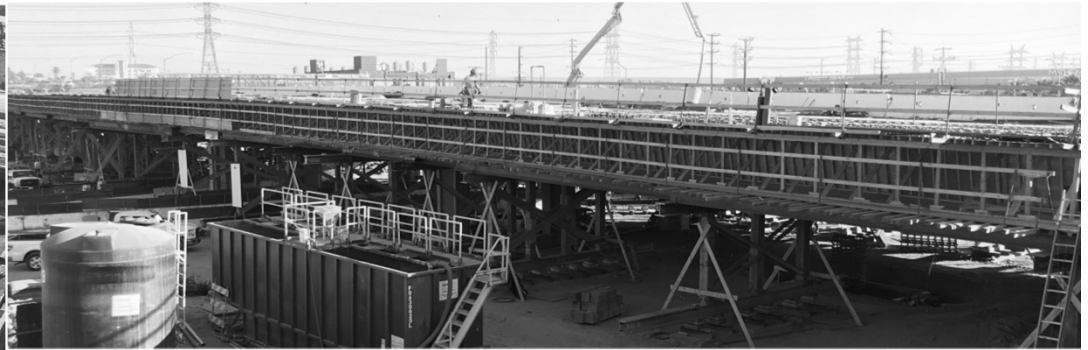
Falsework – Left Side
