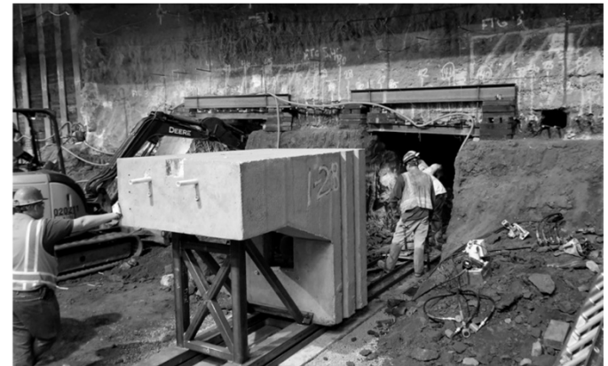
Underpinning activities underway at Historic Broadway Station
