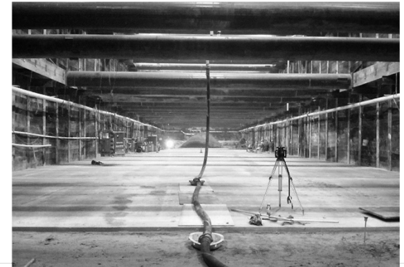
Mud Mat Installation at Wilshire/La Brea Station
