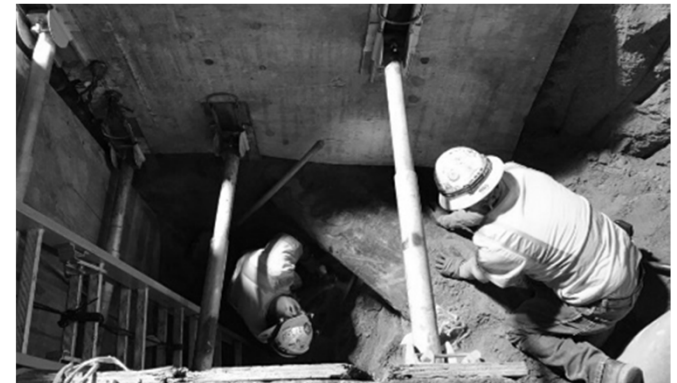
Excavation of 20" waterline on Central Avenue
