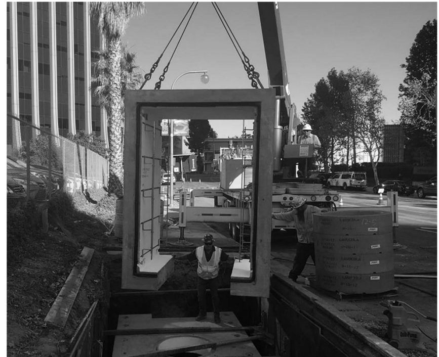
AT&T CA manhole Installation in Century City
