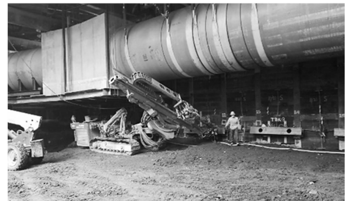
Tieback installation at Historic Broadway Station
