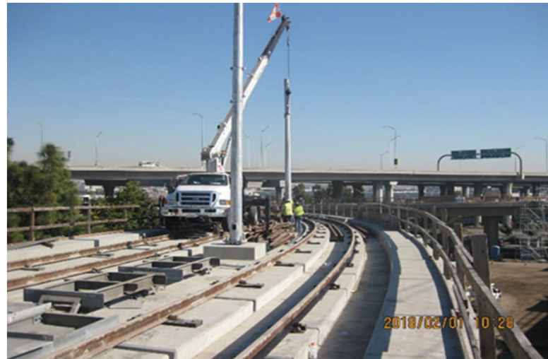
Setting overhead catenary system poles – south end
