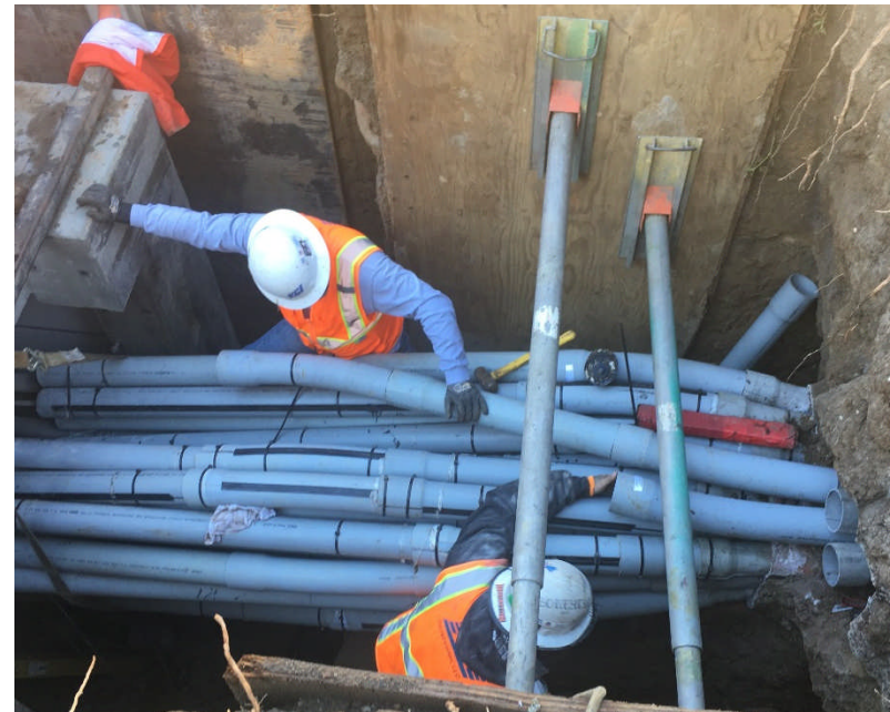
AT&T Conduit Installation in Century City
