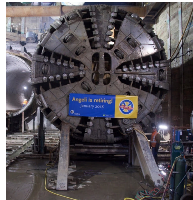
Tunneling completed January 16, 2018
