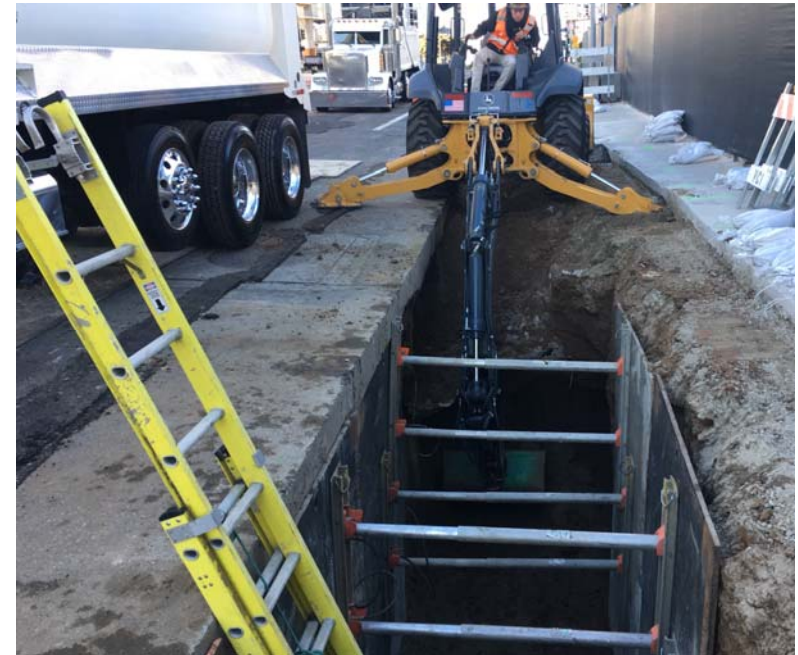
AT&T Conduit Installation in Century City
