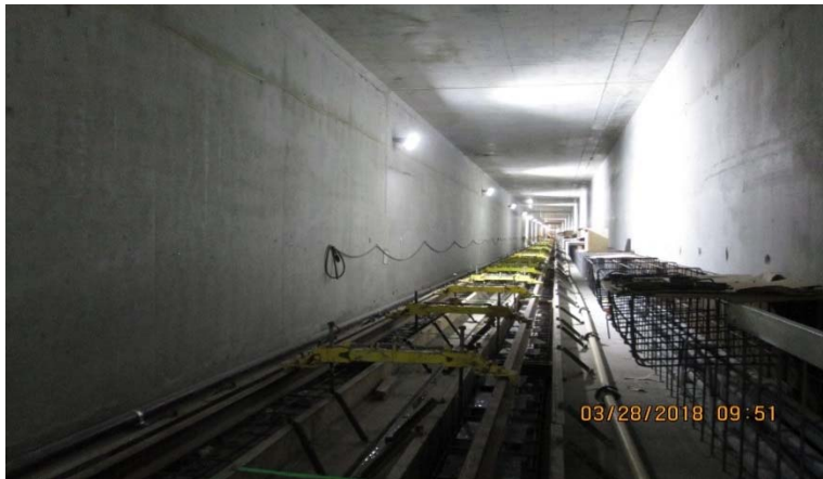
UG #3 Cut-and-cover tunnel – track work plinth construction Southwestern Yard – south yard track leads & APM columns
