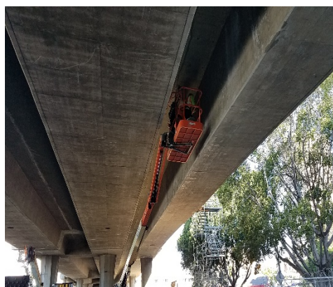
Concrete Finish Work
