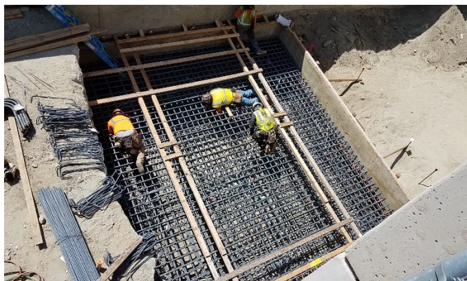
Elevator Footing Forming/Rebar
