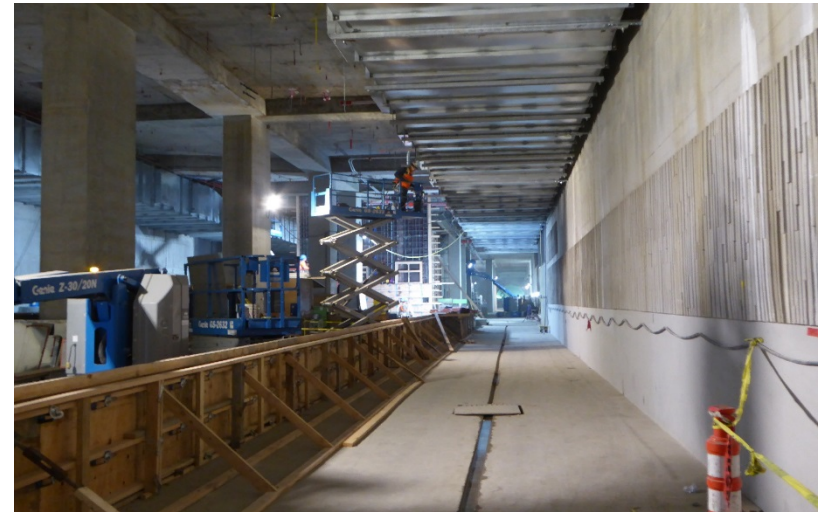
Expo Station; platform area at track level
