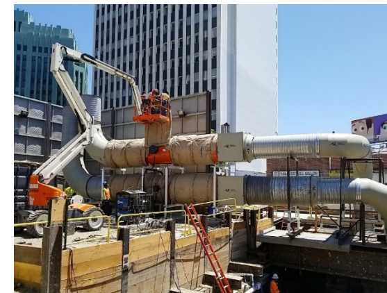
Wilshire/Western Retrieval Shaft
