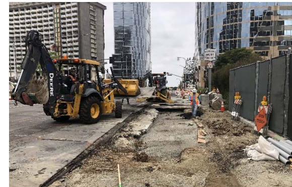
AT&T Utility work in Century City
