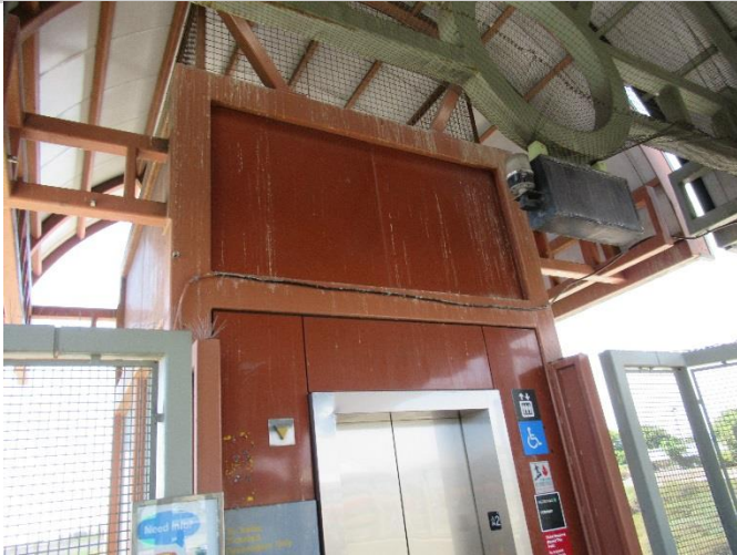
Vermont/Athens Station - Before
