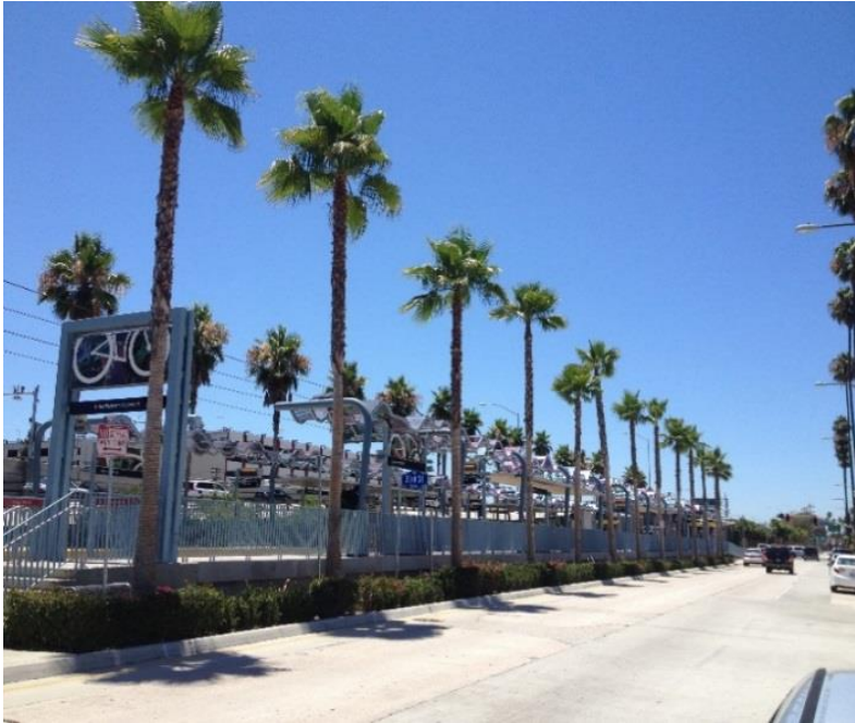
Jefferson/USC Station – Trash Free & Trees Trimmed
