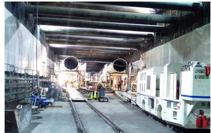
TBM at Wilshire/La Brea Station
