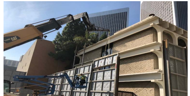
Sound Wall Panel Installation at 1940/1950 Century Park East
