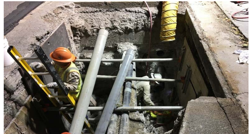
DWP Power Duct Bank and Conduits
