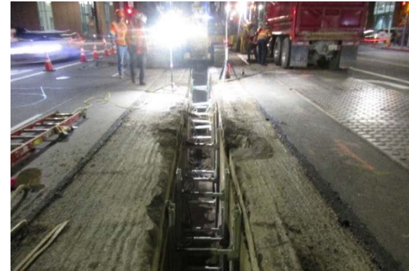
Ductbank Trench Excavation
