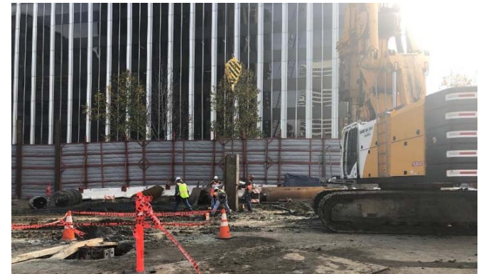
Soldier Pile Installation in Century City
