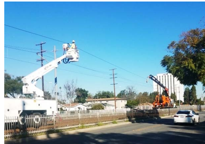
Overhead Catenary System Demolition
