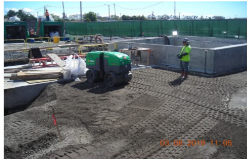
Back filling/compaction of Expo/Crenshaw Station Plaza
