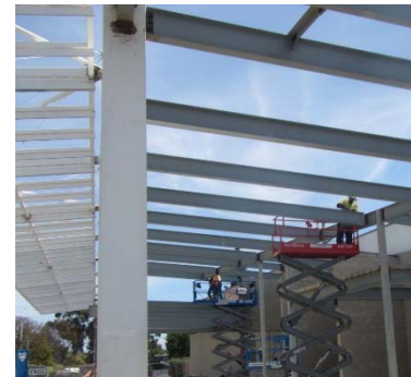
Structural Steel Installation for Mobility Hub
