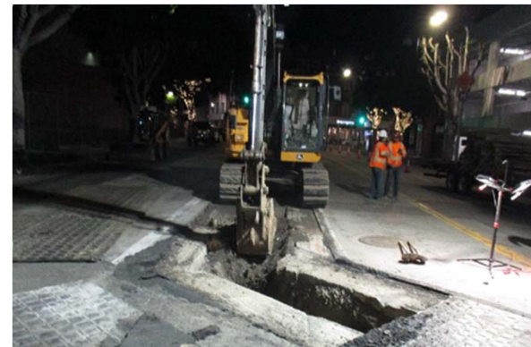
Water Line Excavation and Potholing
