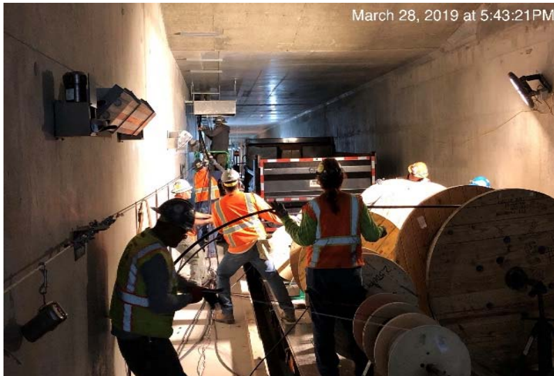
Installing electrical conduit in underground tunnel
