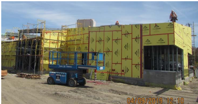
Exterior sheathing at Customer Service Building
