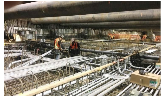
Installation of Conduit at Wilshire/La Brea Station
