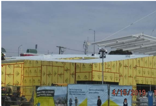
Exterior sheathing at Customer Service Building
