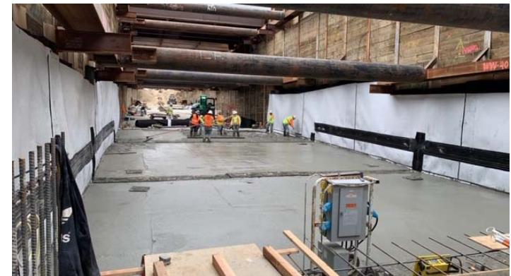
Protection slab placement at 1st Street Leg
