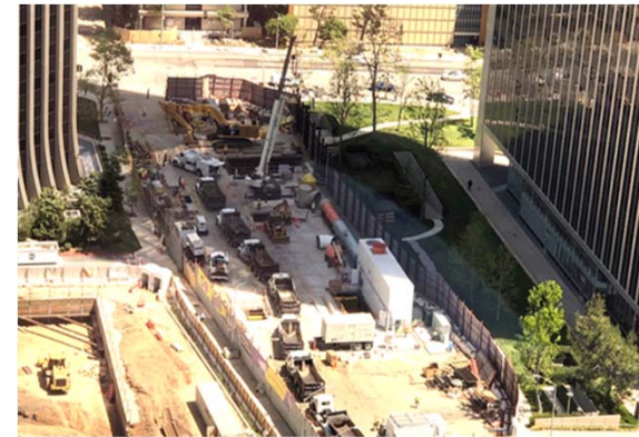
TBM Launch Box Overview in Century City
