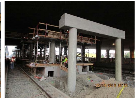
Pile and Beam work at Blue Line Platform/Mezzanine
