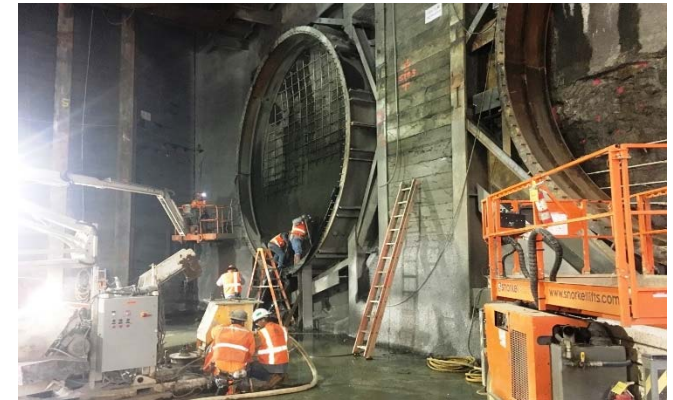
Preparing for TBM Arrival at Wilshire/Western
