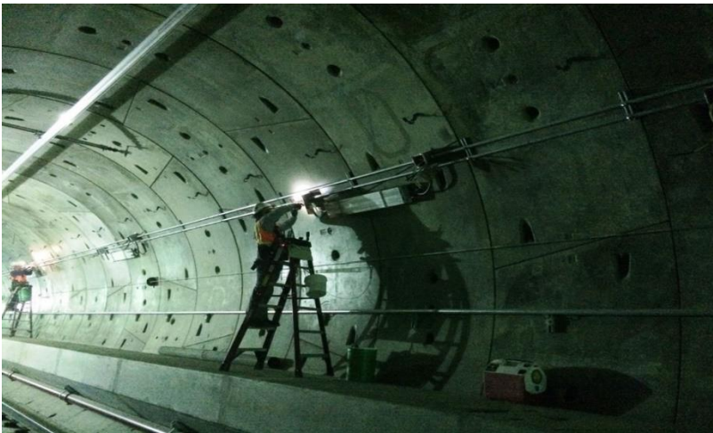
Installation of emergency lighting at southbound tunnel
