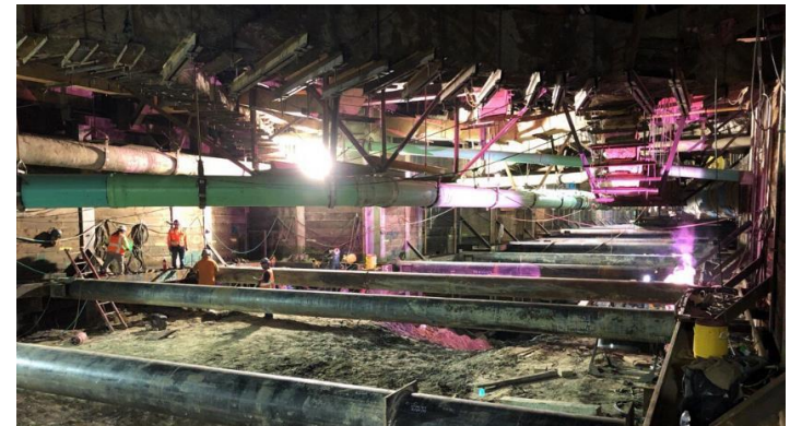
Setting walers at mid-level under Flower St
