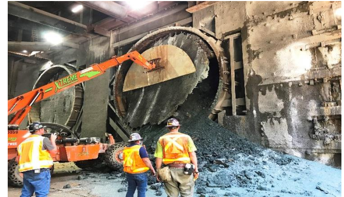
TBM #1 Break Through at Wilshire/Western
