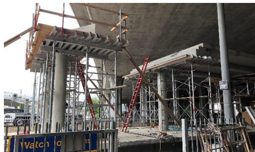
Formwork @ Blue Line Platform/Mezzanine
