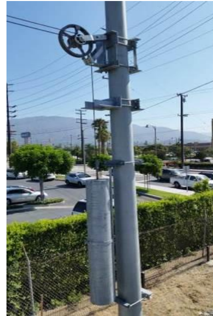
Figure 15: Existing weight stack tensioning system
