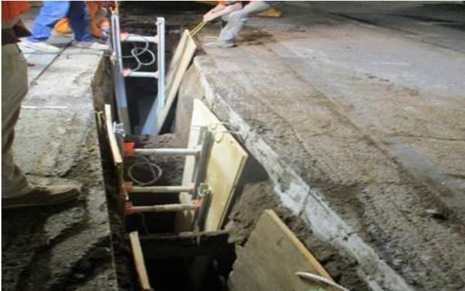
Hand Dug Excavation for Fiber Optic Conduit
