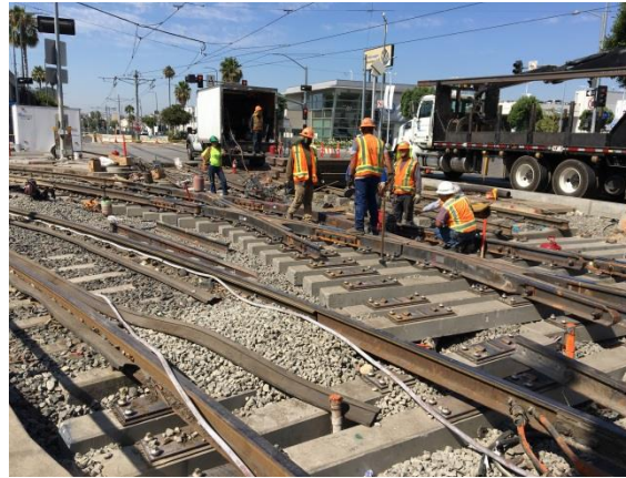
Replacing trackwork at Expo Junction
