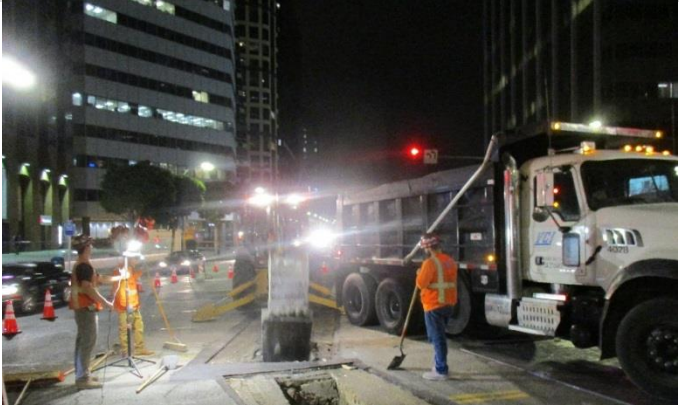
Main Line A Excavation and Potholing
