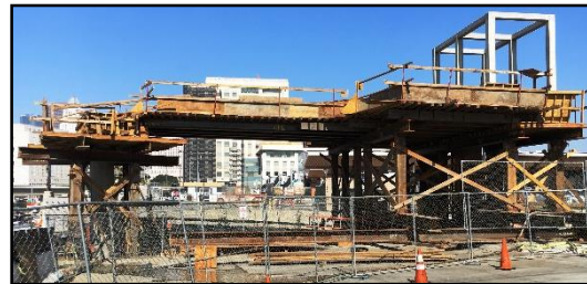
Elevator Platform Falsework
