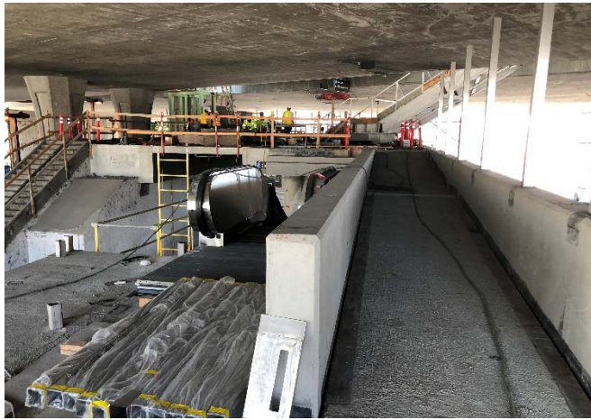
Mezzanine Extension and Platform Work ongoing
