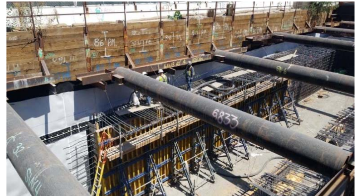
1st Street Cut/Cover Walls pour preparation
