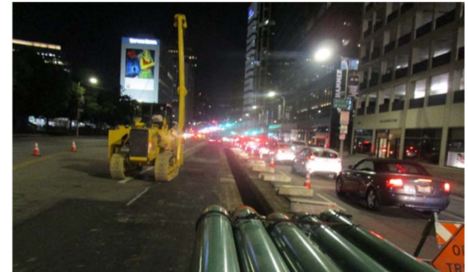
Southern California Gas Steel Pipe Installation
