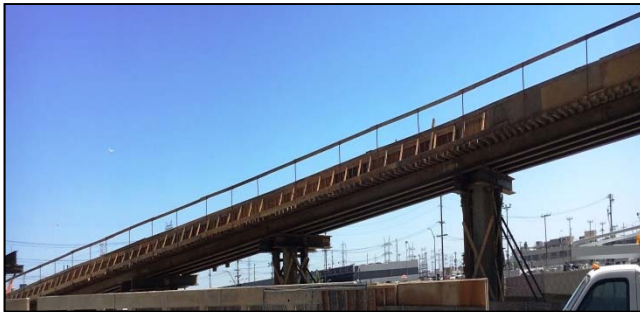
Pedestrian Walkway False work
