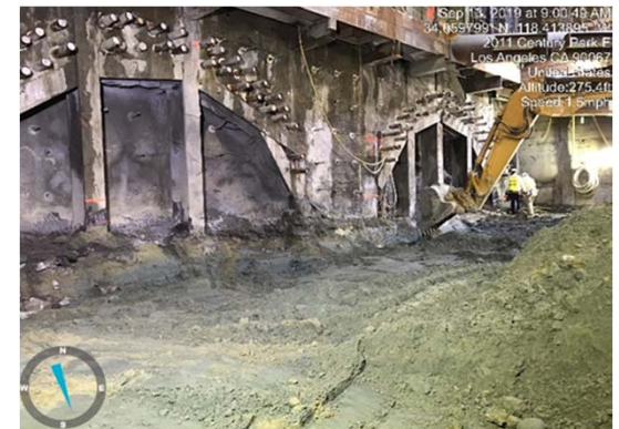
TBM Launch Box Excavation in Century City
