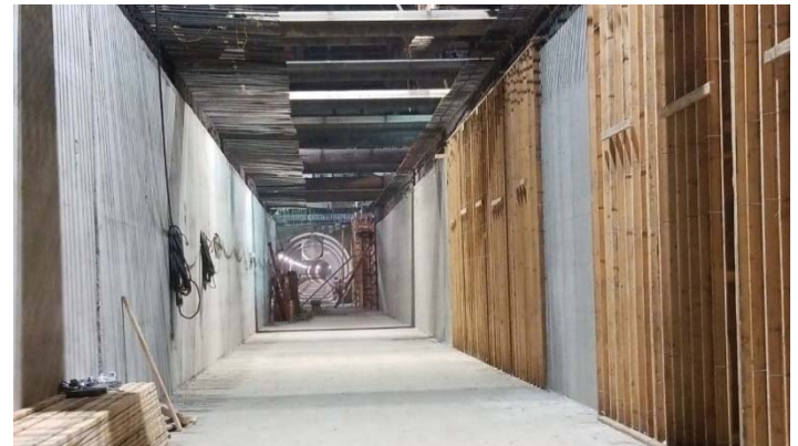
Left track tunnel at Flower St
