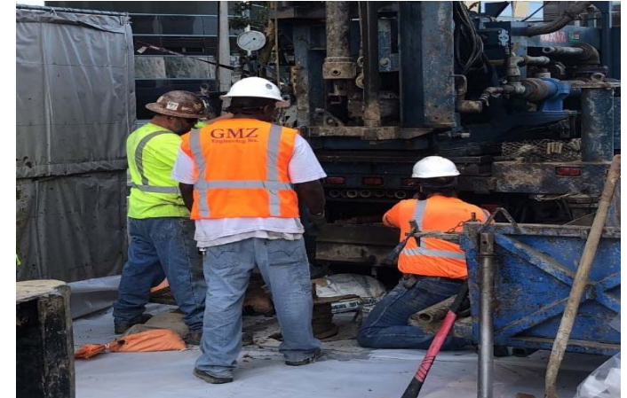
Geotechnical Boring for Tunnel Cross Passage Design at Westwood/UCLA Station
