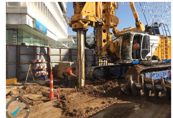
Wilshire/Rodeo Station Box Pile Installation
