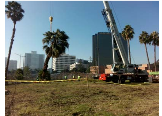
Tree Removal at VA Site
