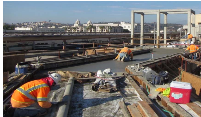
Pedestrian walkway and overcrossing poured
