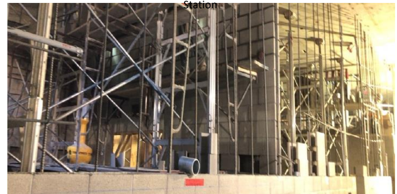
Conduit installation at CMU walls
