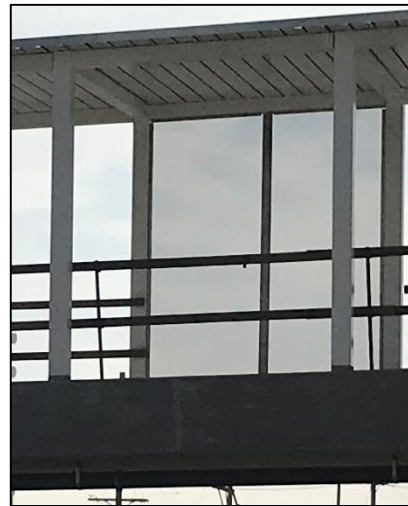
Interior panels initiated
