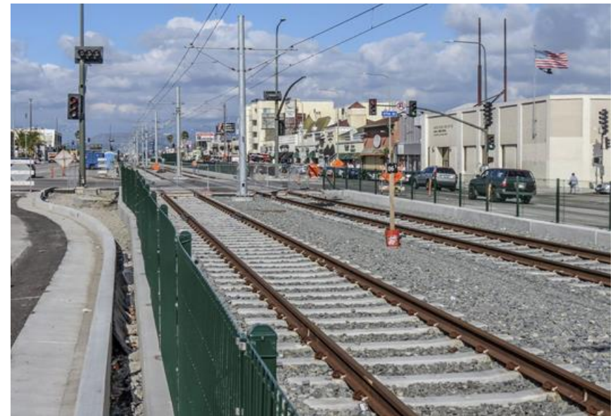
Trackwork and overhead catenary system – Crenshaw & 57 th
