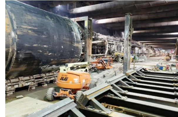
Purple TBM at Wilshire/Fairfax Station
