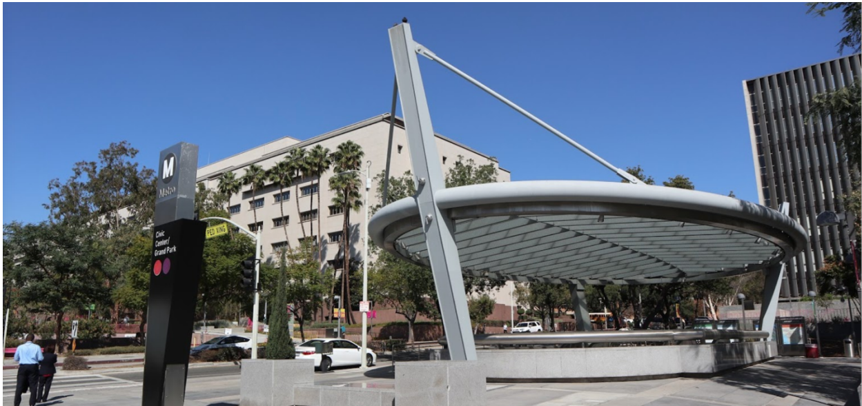
Figure 4.5.1 Civic Center/Grand Park Station
