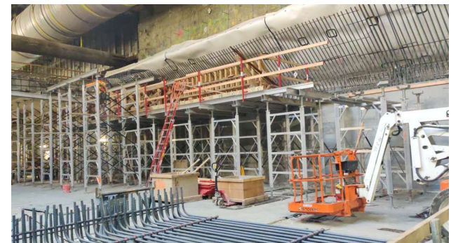
Roof deck shoring installation at Historic Broadway Station
