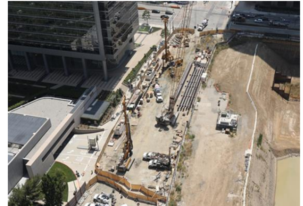
Pile Installation West of the Launch Box in Century City
