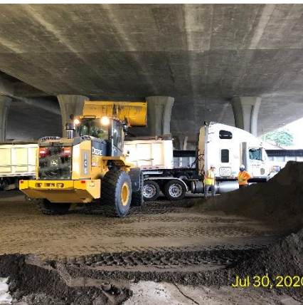
Grading Work @ Package B
