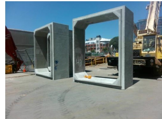
Reinforced Concrete Boxes for Storm Drain Relocation
