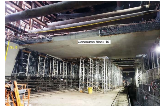
Wilshire/Fairfax Station Concourse Concrete
