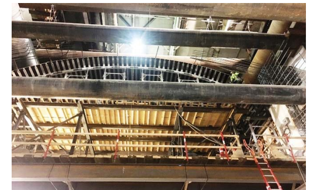
Roof Shoring Frames at Wilshire/La Cienega Station
