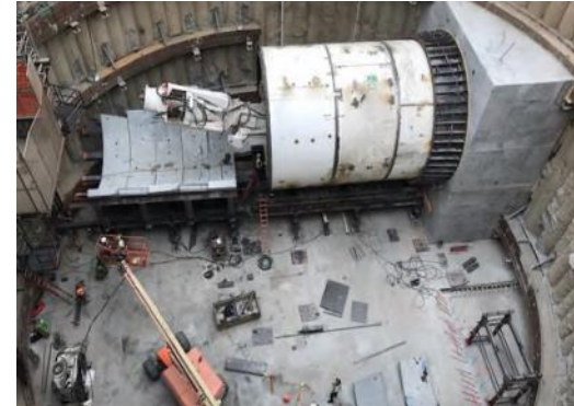
Installation of Temporary Invert Segments on Gantry Cradle at Base of Excavated Tail Track Exit Shaft
