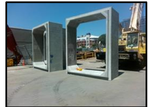
Reinforced concrete boxes for storm drain relocation.
