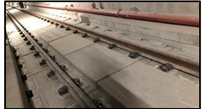
Direct Fastener plates and track assembled in left tunnel reach 2
